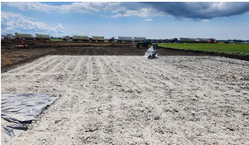
In-Situ Soil Stabilization
