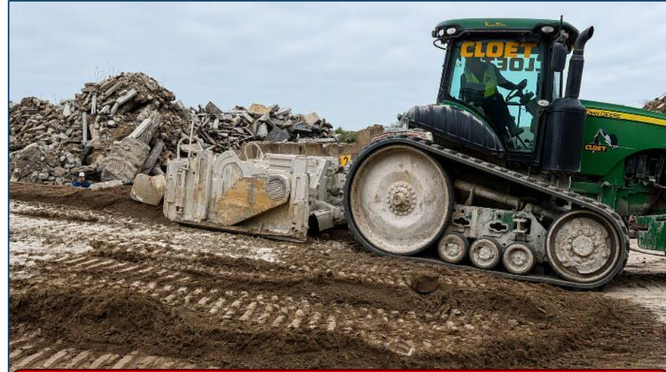
Till into the Soil with Mixing Head
